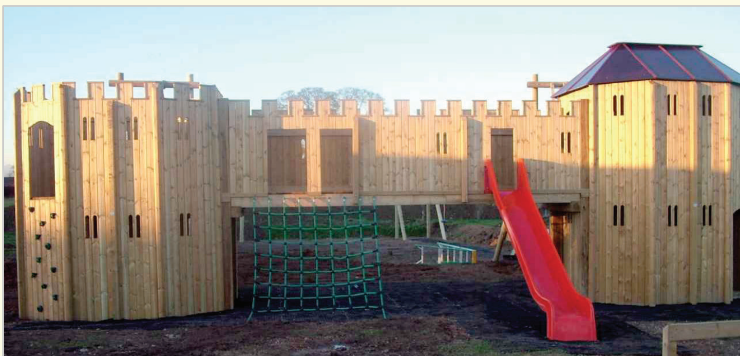
Bspoke Turret and Tower with 6m long bridge, 2m platform height.
